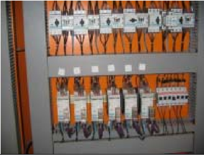
Figure 2: Panel detail – intelligent relays
