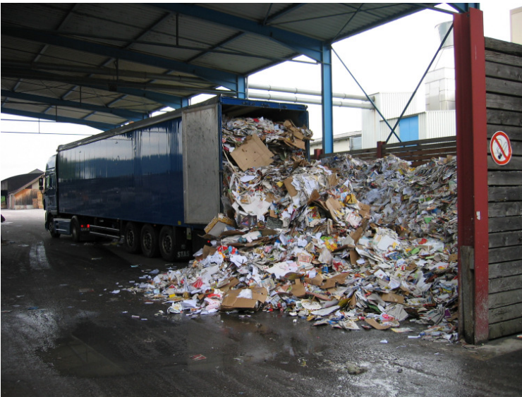
A German Paper Recycling Plant Optimizes Its Energy Usage With A Profinet-based Architecture By Shutting Down Unnecessary Systems During Peak Times
