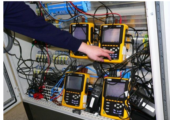
Figure 3 – Measuring setup of PROFlenergy
